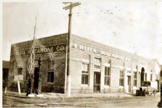
Ferlita Macaroni Factory in 1929 and today as TMD Windows & Doors
